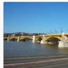
Margaret Bridge 638 m
