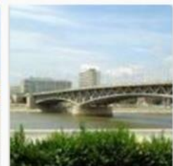
Petöfi Bridge 378 m
